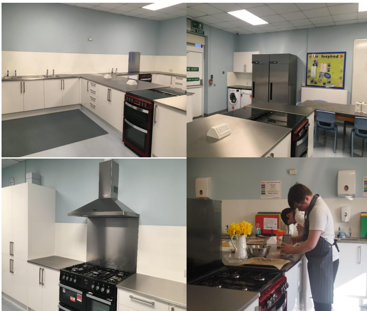
Refurbished teaching kitchen at Cornfield School
